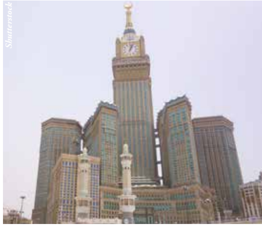
The Makkah Royal Clock Tower Hotel, with a height of 601 m, in Mecca, Saudi Arabia.
