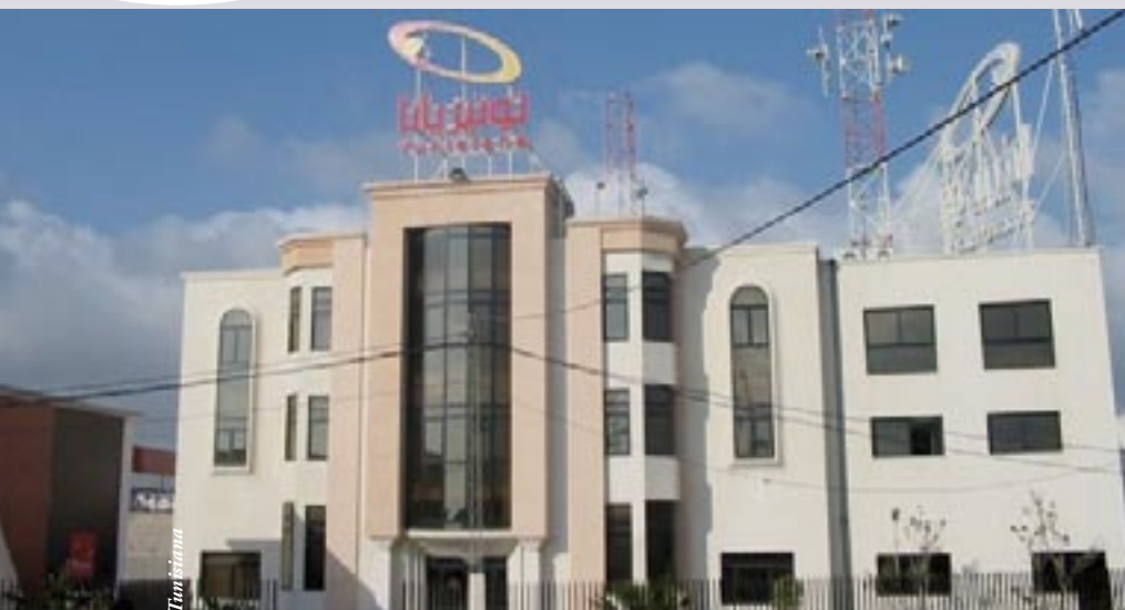
Tunisiana's headquarters in Tunis. The loan will help expand the company's network capacity and finance the final license fee installment.
