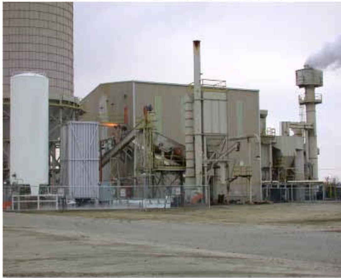
5 MW e CES water cycle plant at Kimberlina, California
